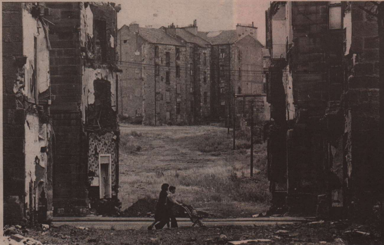
Decay in Glasgow, Maryhill. Photo: John Sturrock, Report.
